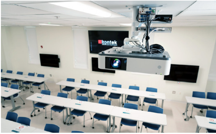
Active learning classrooms have a flexible setup and can be reconfigured to address semester-based pedagogical needs. An Extron NAV E 101 is installed with the PTZ camera over the suspended exam table to send images to the Distance Education Control Room over the UNCW network. This classroom is shown in the traditional configuration, which is better for social distancing.
